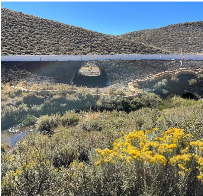
Figure 20: One of the completed junction under crossings.
