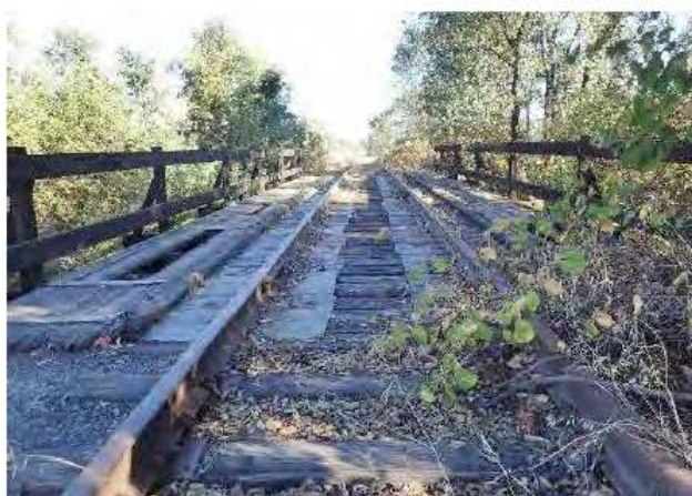
Figure D-4 Deck Plate Girder Bridge at Hensley Creek (MP 116.4), Built in 1913
