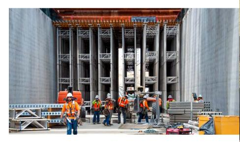
California High-Speed Rail crews assembling scaffolding for the construction of a trench box lid.
