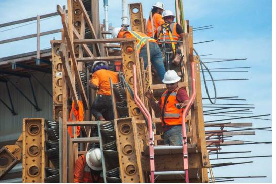
Workers inside the concrete forms constructing wing walls for the Avenue 12 overcrossing.
