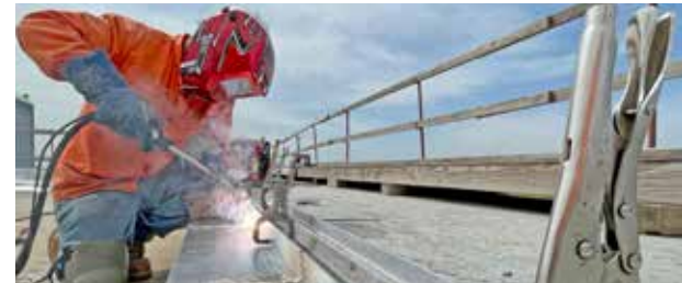
A welder works on the Conejo Viaduct in Fresno County
